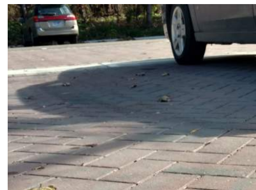
Permeable parking lot bays
